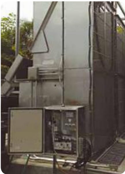
Waste water treatment
